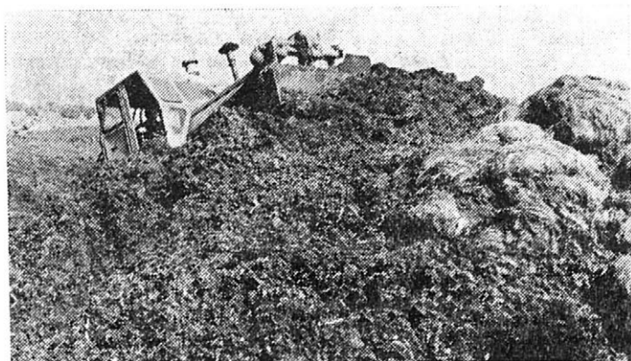
6. Promíchání kompostu buldozerem S-130 — Compost mixing by the S-130 bulldozer
